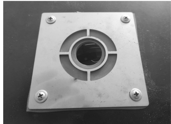
View of exhaust floor plate from below
